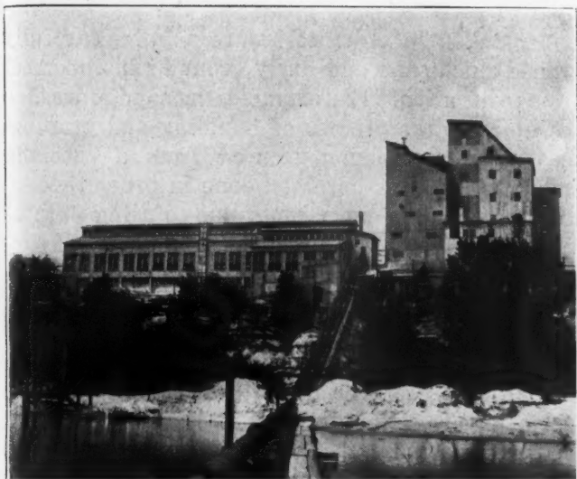
Plant A and Power House
